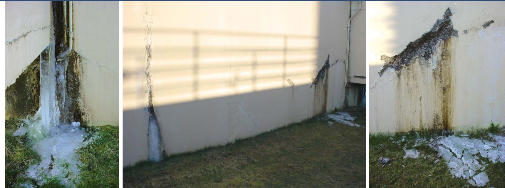
The frozen seepage in these photos highlights the extremely deteriorated condition of the concrete basins, and these freezing conditions have accelerated the deterioration. (December 2009)
